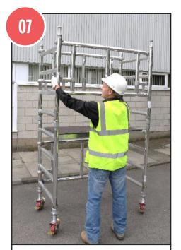
7. Fit a guardrail frame to each side of the platform (hooks facing outwards) Top hook above the top rung of the end frames. (Refer to labelling to ensure that the frame is the correct way up).
