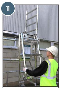
11. Stow the guardrail frames on the front assembly bracket.
