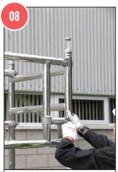
8. Ensure that all frames are securely fitted and that they are located the correct way up (use labelling as a reference).
