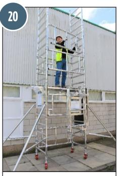
20. Fit 1 side guardrail the 3rd rung above the existing as shown.
