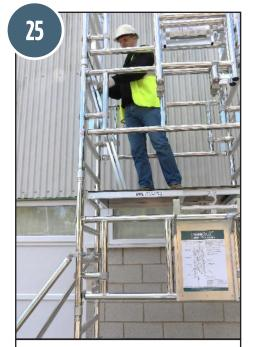
25. Temporarily locate the toeboard assembly on the platform to allow access to the additional platform that is stowed.
