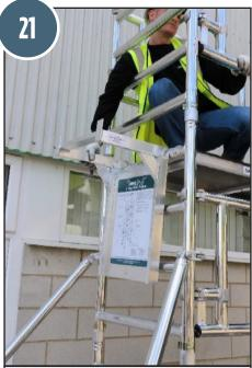
21. Relocate the "empty" assembly bracket from the side of the tower.
