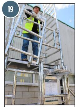
19. Retrieve a side guardrail frame from the front assembly bracket and pass upwards as shown.
