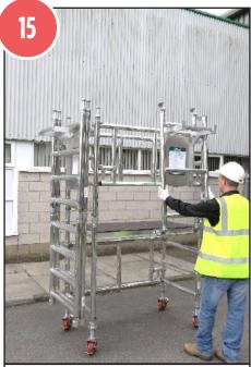
15. Stow 3 guardrail frames on the front assembly bracket.
