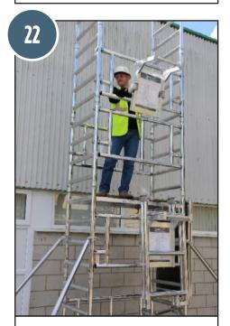
22. Place the removed bracket on the top rung of the tallest guardrail frame as shown.
