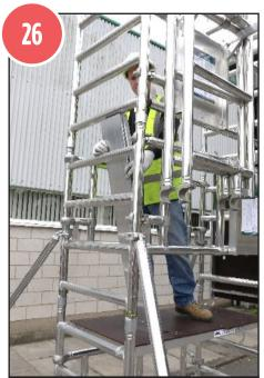
26. Temporarily locate the toeboard assembly on the platform to allow access to the additional platform that is stowed.
