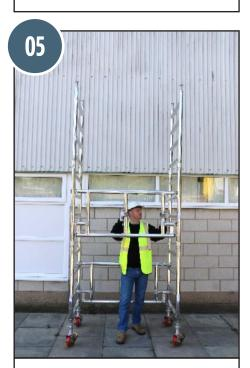
5. Fit 1 guardrail frame above the 7th rung. Hooks facing outwards. (Refer to labelling to ensure that the frame is the correct way up).
