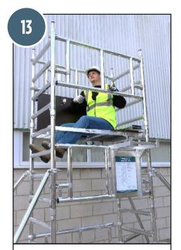
13. Fit 2 guardrail frames, with the top hook (facing outwards) set above the top rung of the frame.
