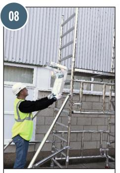
8. Fit an assembly bracket on the side of the tower.
