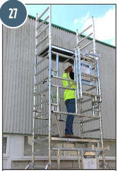
26. Remove the remaining platform from the lower section of the tower and pass up through the side frame.
