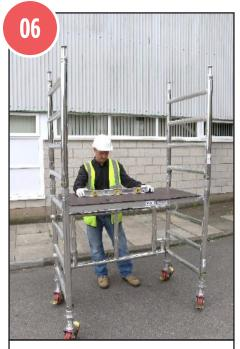
6. Ensure that the tower base is level at this point.
