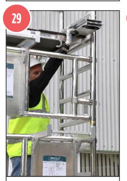
29. Relocate the toeboard assembly from the lower platform to the higher level, ensuring that it is positioned on the plain section of the platform as shown.
