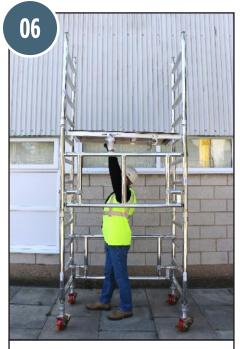
6. Fit the platform, 1 rung above the side frame location as shown.
