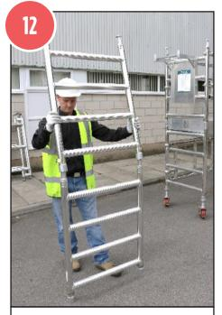
12. Assemble the frames in pairs as shown.
