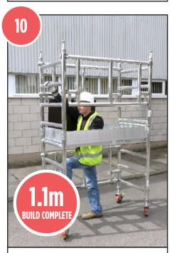
10. Access the platform using the trapdoor as shown and begin work.
