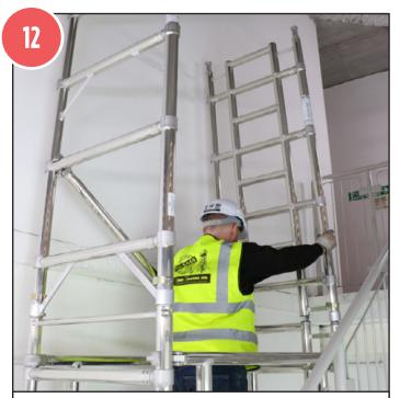
Fit a plain 4 rung frame to the ladder portal frame and engage the interlock clips.
