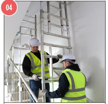
Position the ladder portal at the bottom of your stairs and connect the horizontal braces above the 3rd rung. Level the tower by adjusting the legs.
