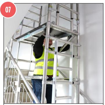
Fit a platform to the 3rd rung of the plain portal frame, trapdoor at the ladder frame side.
