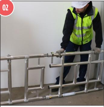
Fit the offset ladder frame\* on to the ladder portal frame & position the frame down the stairs.
