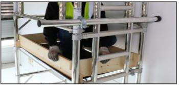
Fit a side prop to the top of each frame, one either end of the tower and then fit your Toe-boards to the tower using the clips.
