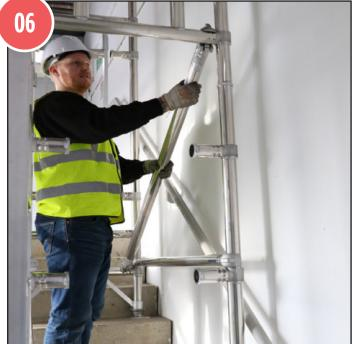
Fit another diagonal from the bottom rung of the plain portal frame to the top rung of ladder portal frame on the right hand side.
