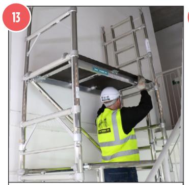
Fit a platform to the 2nd rung of the 4 rung plain frame with the trapdoor on the ladder frame side.
