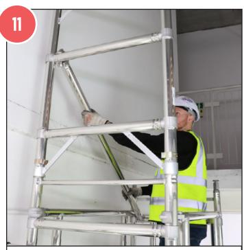
Fit a diagonal brace from the 2nd rung above the platform to the second rung of the 4 rung plain frame.
