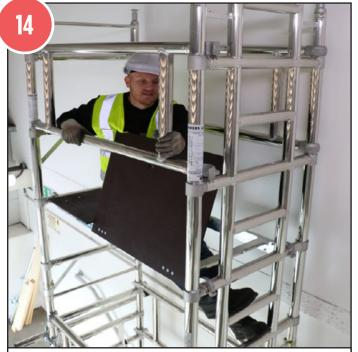
Sitting through the platform, fit 2 guardrail frames, one either side or 4 Horizontal braces 2 either side with hooks facing out. Repeat steps 1 - 5 to build additional heights
