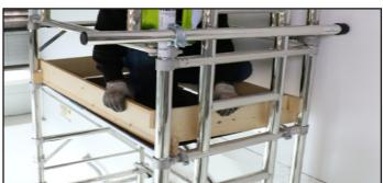
Fit 2 side props every 2m, one either end of the tower. If you cannot fit side props, stabilizers shall be fitted to all 4 corners of the tower. They shall be fitted to create the largest footprint possible. Then fit your toe-boards using the clips.
