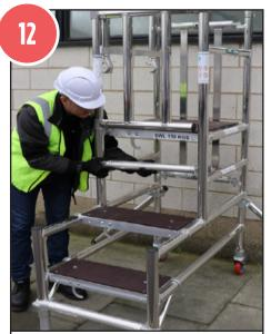
Add the additional brace below the platform. For a stepfold 2 you should now have 2 ribbed braces below the working platform.
