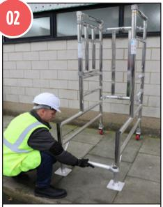
Fit a ribbed brace above the lowest collar as shown.
