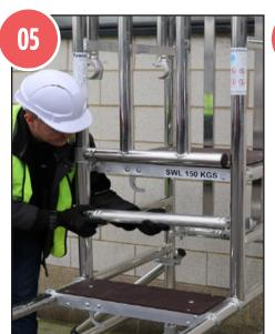
When building the Stepfold 2 add a ribbed brace below the platform.
