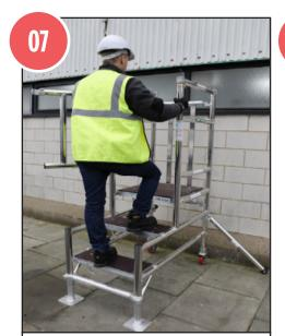
Ascend to the platform using the step platforms and ribbed brace.
