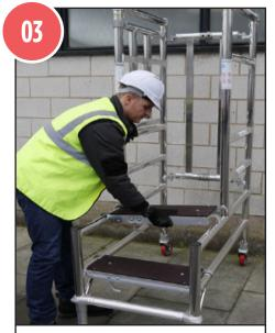
Fit the step platforms on the 1st and 2nd rung as seen above.
